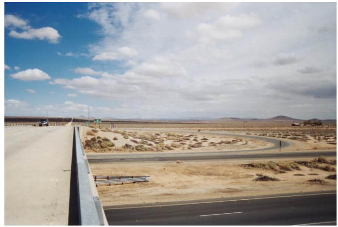
Photograph of Interchange Ramp (east of parcel) onto Westbound Highway 58
